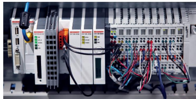
The DeltaBot line was recently upgraded with Beckhoff CX1010 Embedded PCs running TwinCAT PLC software to boost controls performance while reducing cost.
